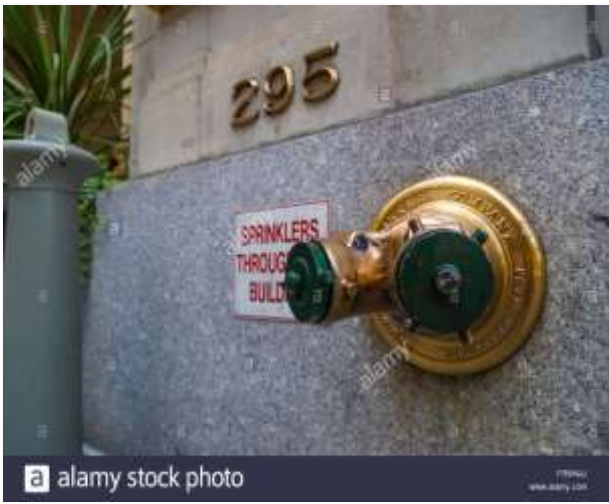
FIRE HYDRANT SPRINKLER CONNECTION IN A WALL
